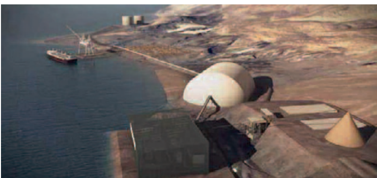
3D-model of the shipment, storage and process plant facilities to be constructed in connection with a mining operation at Citronen Fjord (Ironbark Zinc Limited).
