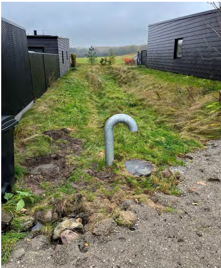
Infiltration trench with overrun pipe from upstream ponds and trenches
