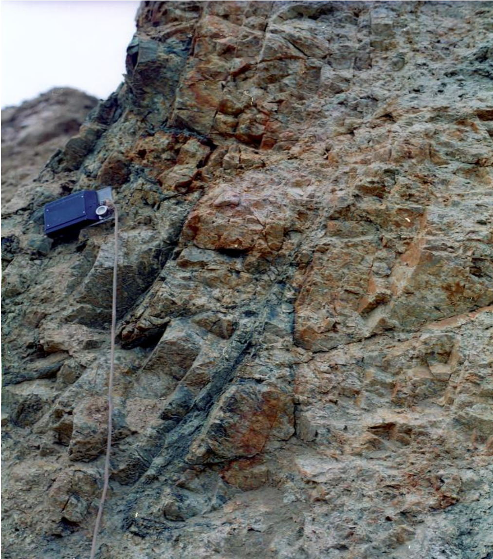
Figure 47. The presence of subvertical fractures and faults in Almindingen Granite. Diabase dykes is associated with weathering of the rocks and the diabase is often altered to greenish clay.
