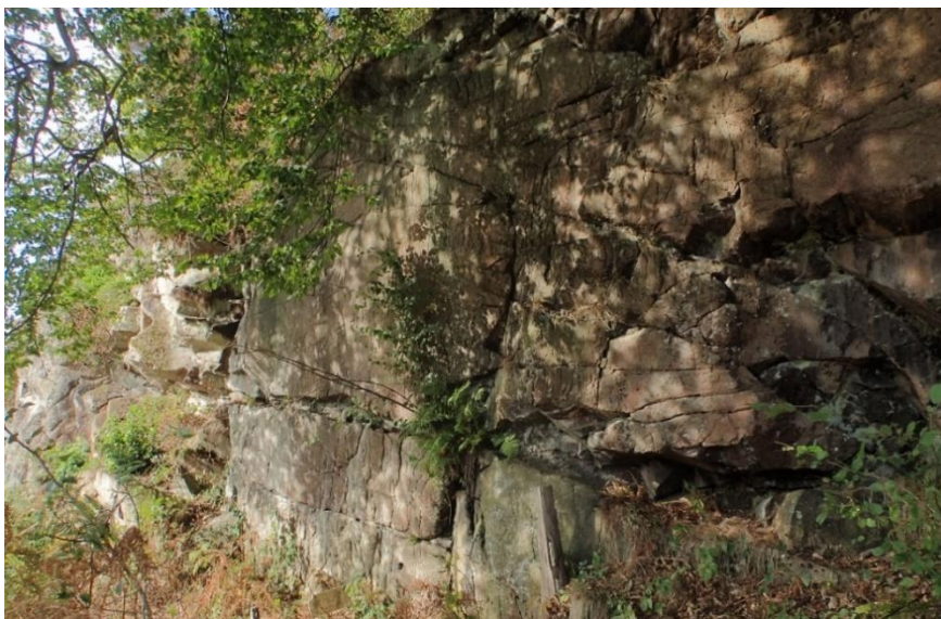
Figure 46. Picture showing a close-up of the fracture seen on Figure 45. It occurs as a several cm wide, sub-horizontal fracture in the central part of the picture and is associated with several minor fractures.
