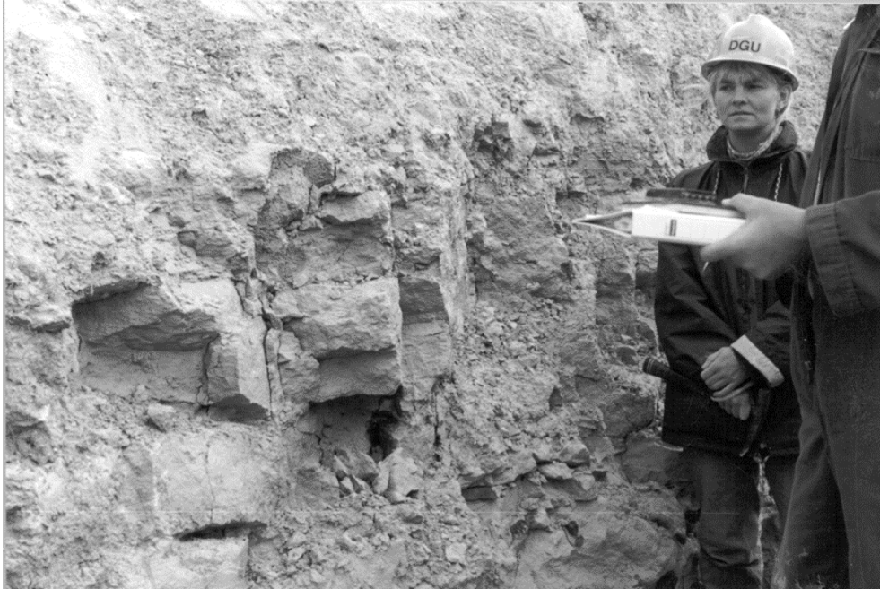
Figure 23. Vertical fractures in the København Limestone Formation in a temporary exposed outcrop in København.
