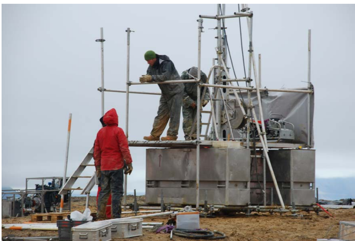
Figure 2.2. Assembling the drilling rig.
