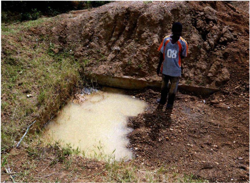
Fig. 8-4. Concrete-lined basin for washing eluvial material containing spessartine. The fine-grained material deposited in the basin is prevented from being washed into the drainage system.
