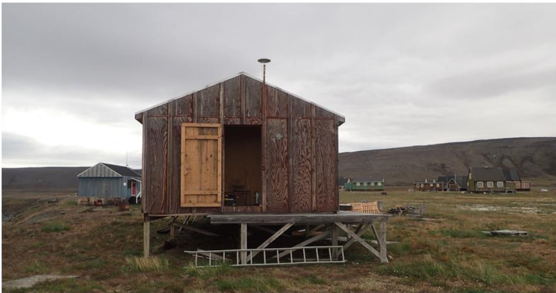
Figure 5. The base antenna mounted onto a house in Moriusaq.
