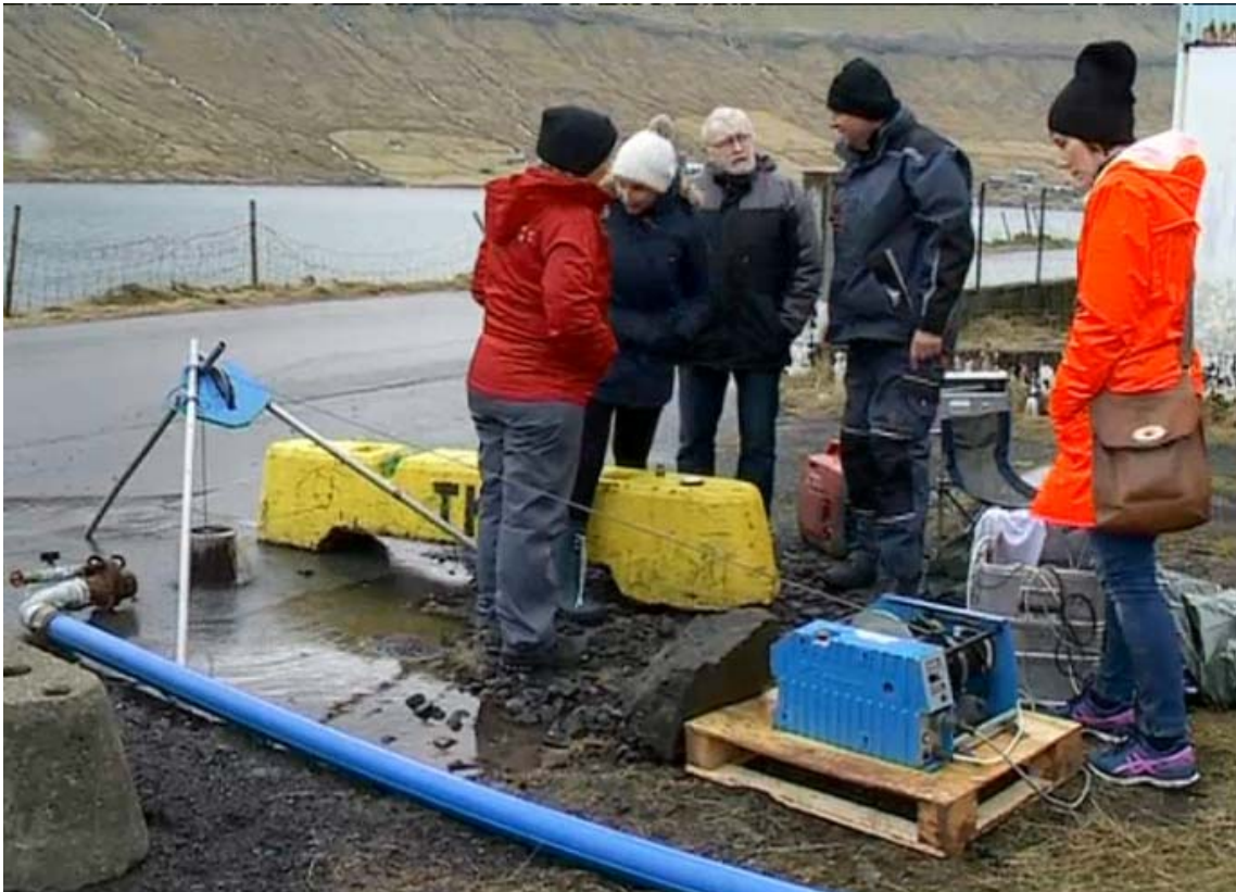
Figure 2-1. Photo showing winch, cable and shear legs from logging borehole UB1 (from “kvf.fo broadcast 25.01.2016 - 20:04”)
