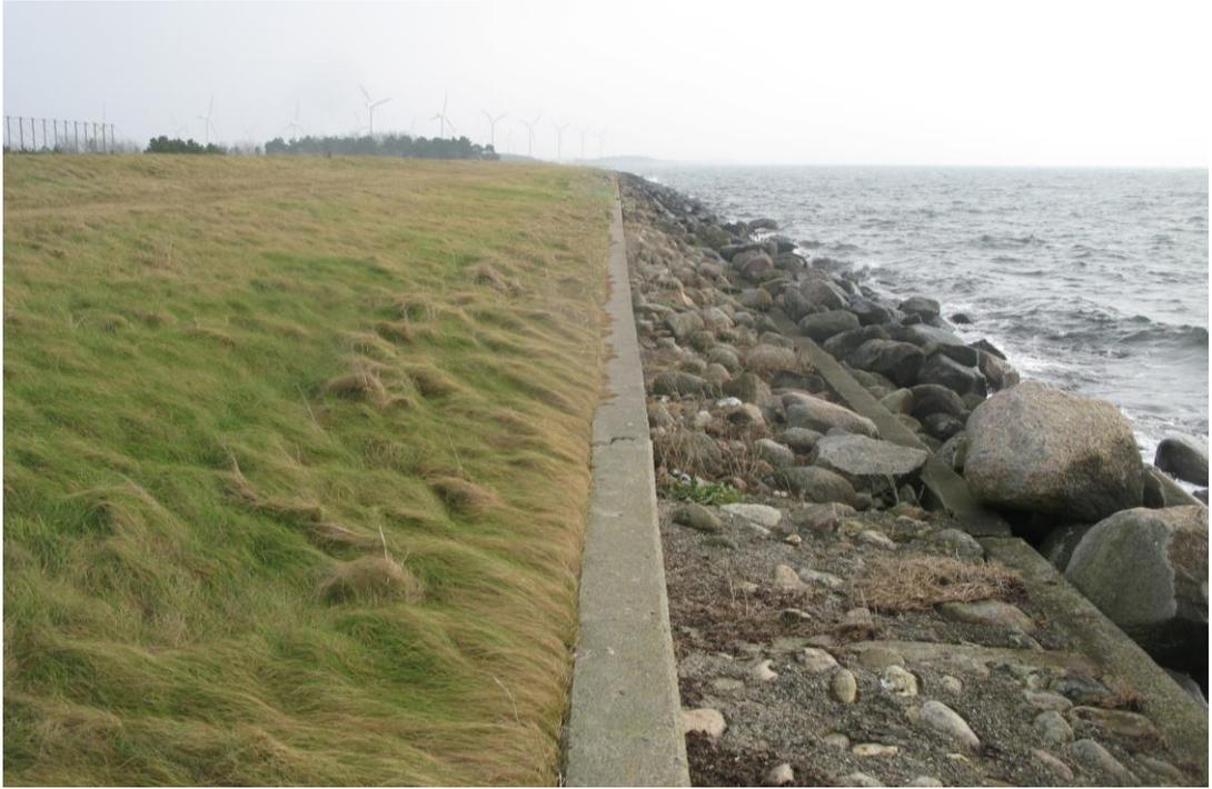
**Fig 16.** Along the Baltic coast the foot of the dike is reinforced along long stretches.
