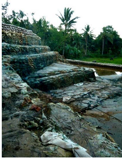
Figure 3. Large heap of mine tailings "secured" with deteriorating plastic bags filled with tailings.
