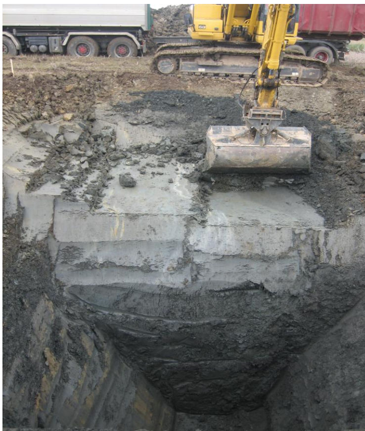
Figure 6. Excavated profile in fine-grained clay from the Holmehus/Ølst Formation (From Gravesen & Pedersen, 2009).
