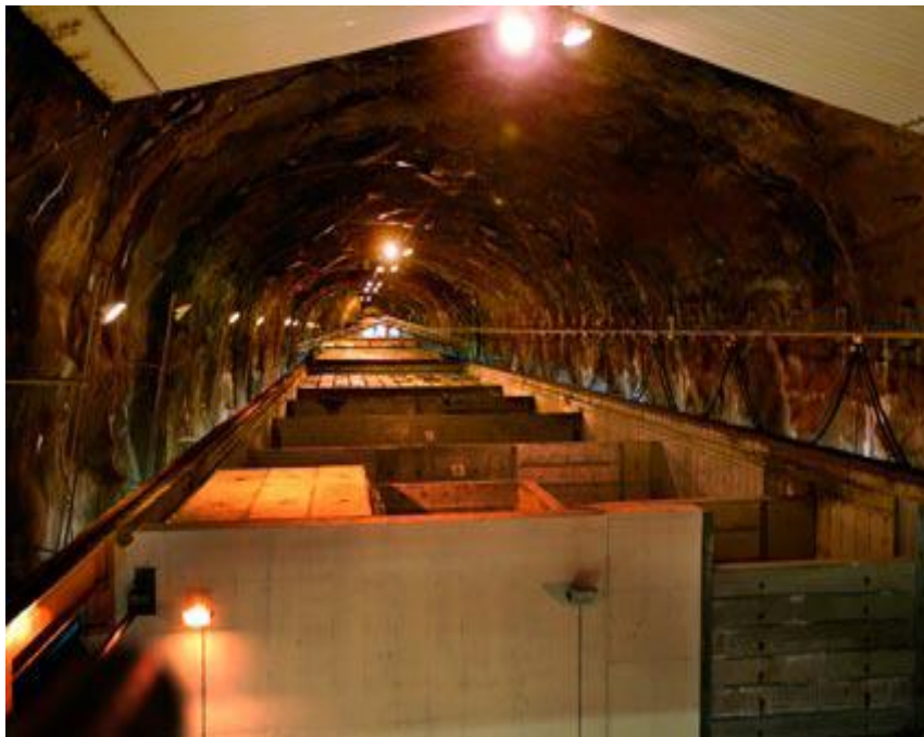
The interior from the final repository for low- and intermediate-level operational waste at Formark, Sweden (From SKB, 2007). The waste is deposited in a rock cavern without shielding in Precambrian basement.
