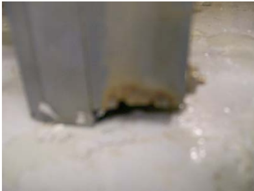
Figure 10. Bottom of the float structure of OBS D after it was damaged by a wave.
