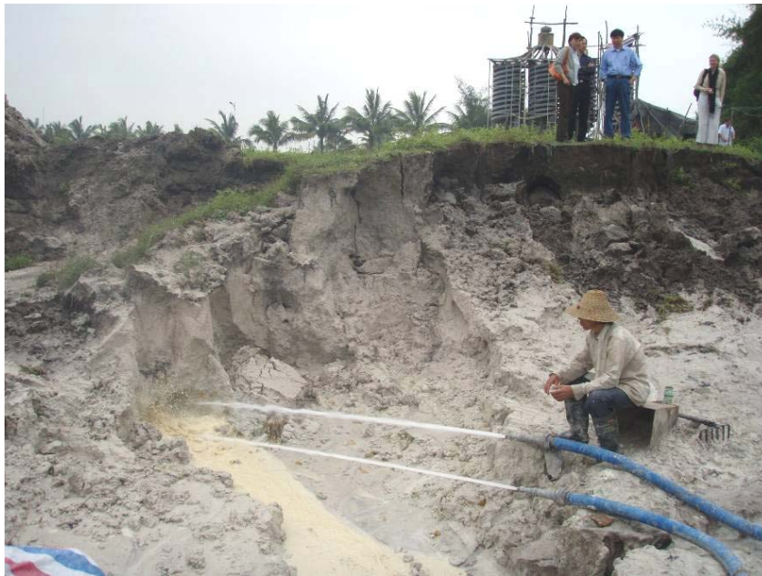
Figure 6. Water hoses responsible for producing slurry for the spiral concentrator.
