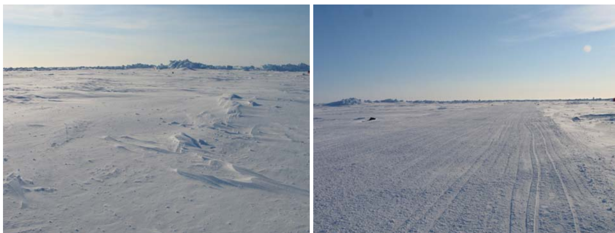
The runway before and after grooming with the bunk drag
