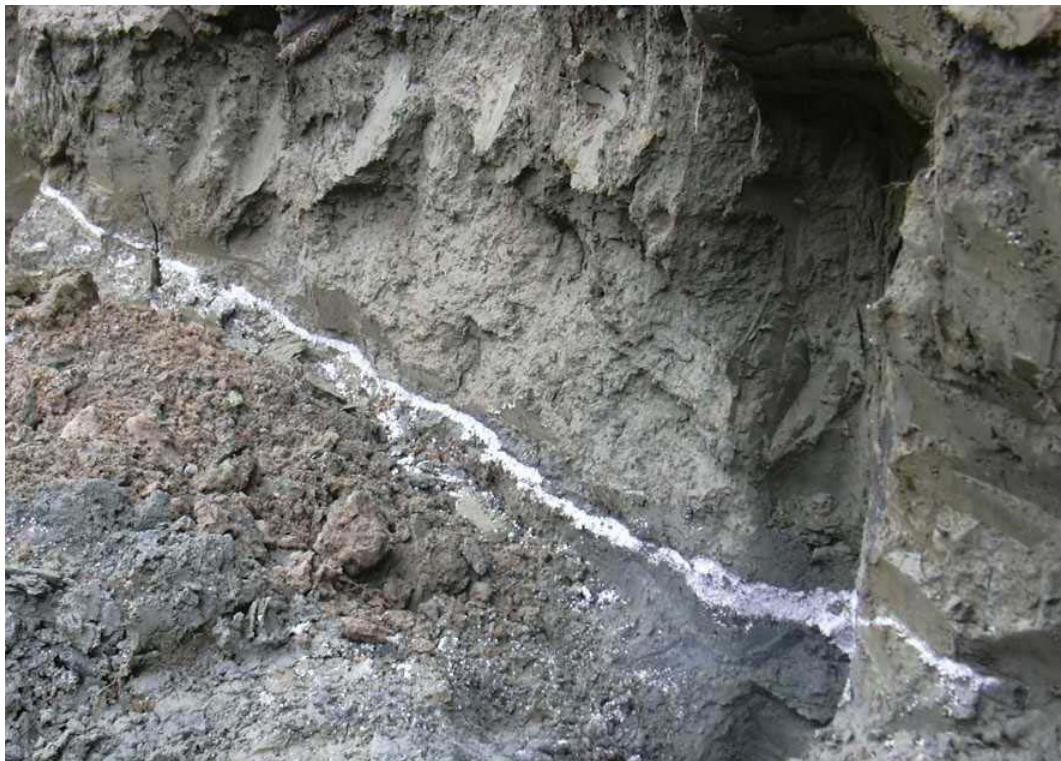
Figure 19. Excavation of Cell 5, where the Mickey Mouse ear procedure was trained (See text). The photo shows an almost horizontal white sand-filled hydraulic fracture at 2-2.5m depth. The width of the white coloured sand fracture varies between a few mm to 5 cm.
