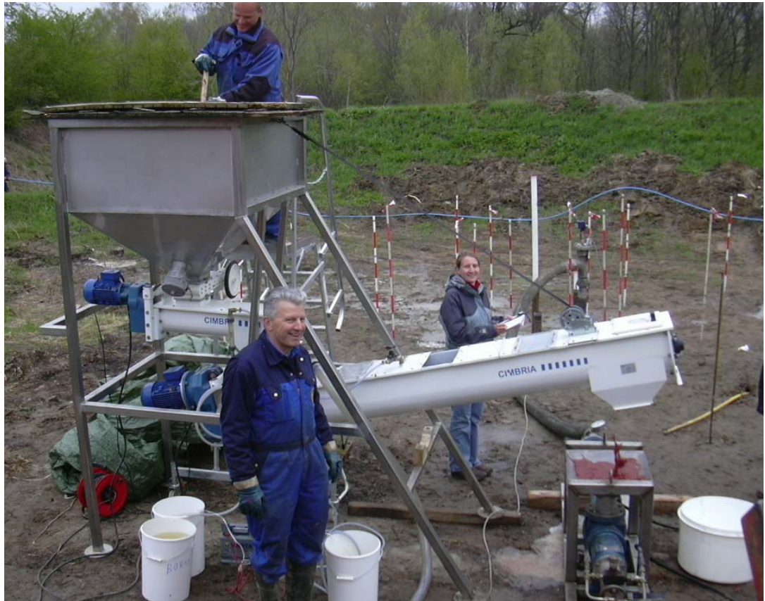
Figure 2. Mixing equipment with tower for sand mixing at the left and in the middle a fully adjustable electrical feeding and mixing auger
