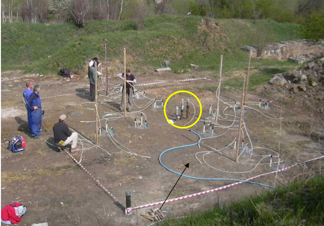
Figure 8. Field instrumentation of Cell 2 for pneumatic tests (see also Nilsson et al, 2006b). Yellow circle: Fracturing wells at 2.5 (left), 3.5 (mid) and 4.5m (right). All other white plastic pipes are monitoring wells for hydraulic testing. Arrow points to the North.
