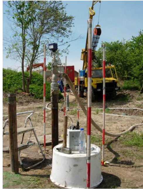
d) 2 inch hose to injection wells
