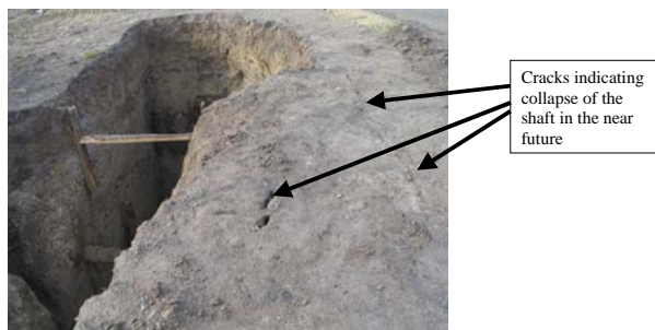
Figure 7. Cracks near a shaft. These cracks indicate that there will be cave in of the walls in the near future.
