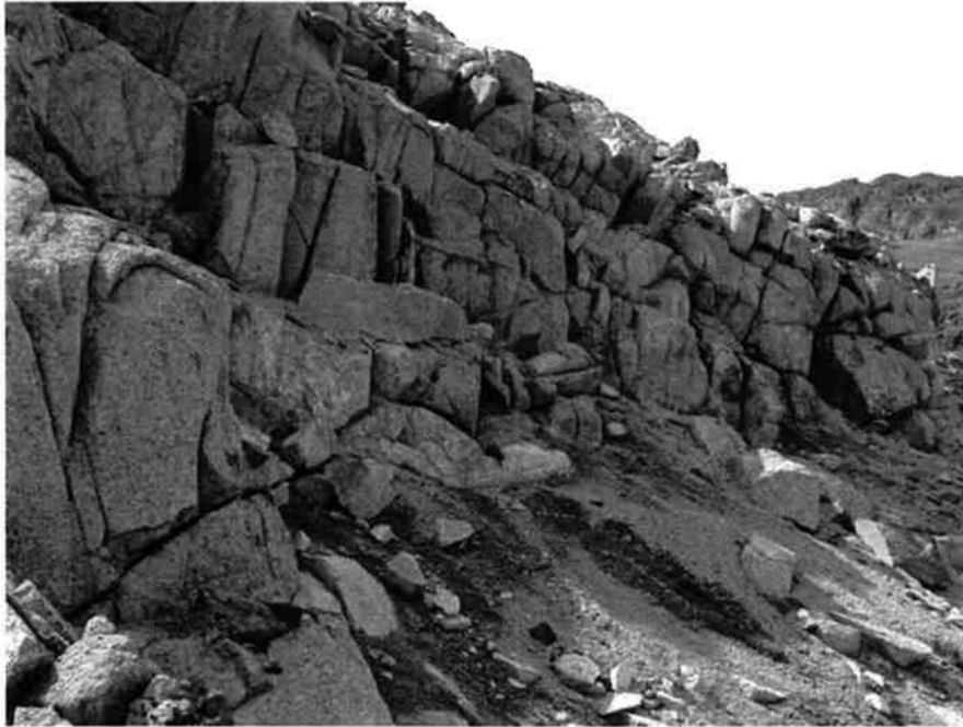
Figure 54. The syenite at Tuttutooq is strongly weathered and many tight joint in several directions.
