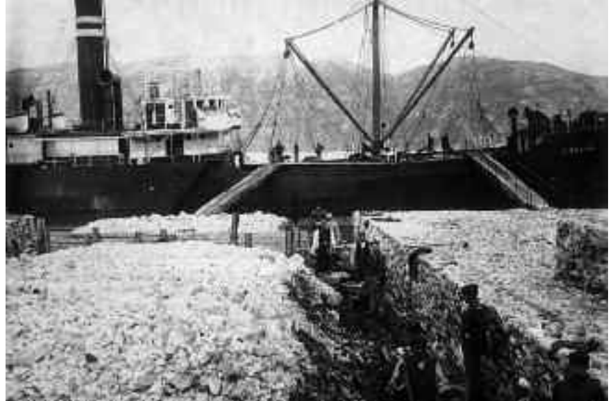
Large piles of well-sorted cryolite ore in the process of being manually loaded onto the ship Thelma at the Ivittuut Cryolite Mine (1920) in South Greenland. The open pit mine was active from 1854 to 1987.
