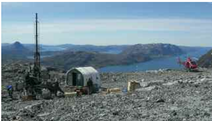
Drilling at the Kvanefjeld multi-element deposit in 2011. Photo: Greenland Minerals and Energy.
