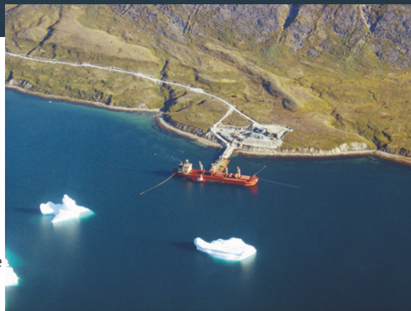
A docking bulk-carrier at the Nalunaq port. Close to the pier is the location of the ore storage facility with a number of ore piles. The road connection to the Nalunaq mining camp can be followed along the coast line.
