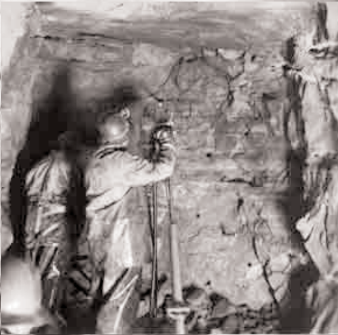
Drilling. Photo: GEUS.
