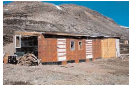
Improvised housing built of beer boxes at Nyhavn. Photo: Niels Pugholm, 'Blyminen i Mesters Vig', published by Atuagkat, 2005.
