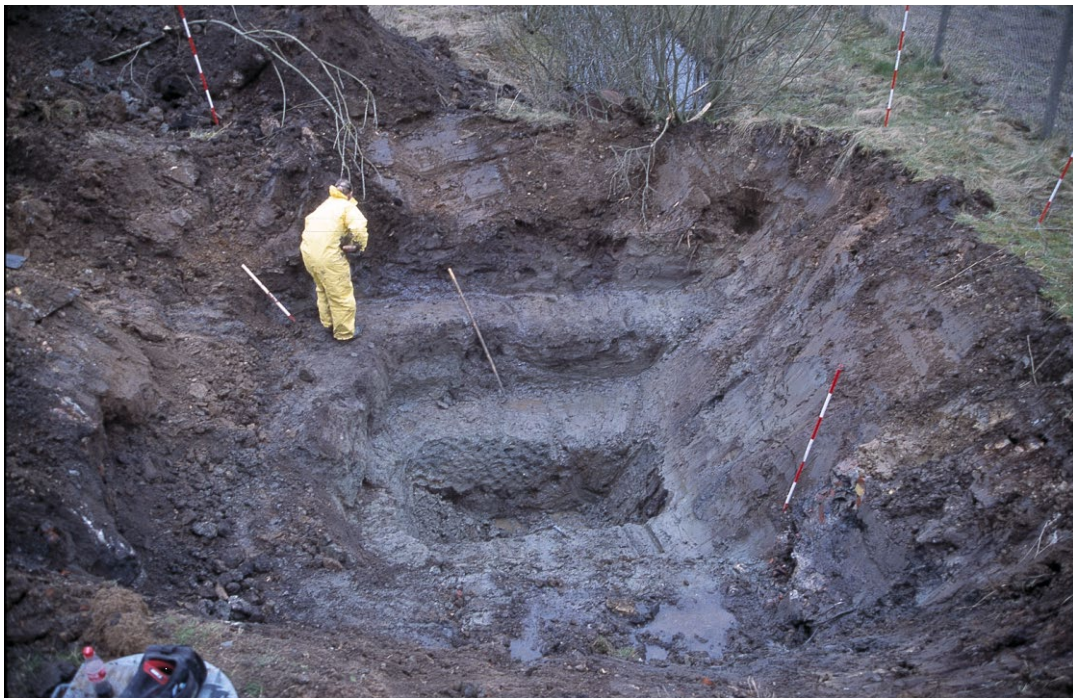
Figure 5.1 Pit no. 4. All matrix was saturated with dissolved phase contamination.
