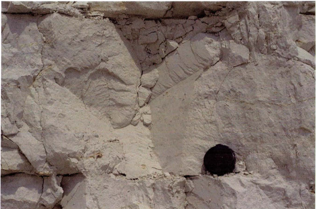
Figure 15. Fracture surfaces associated with the smooth vertical fractures.
