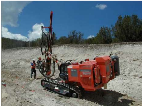
Fig. 4 Percussion drill rig
